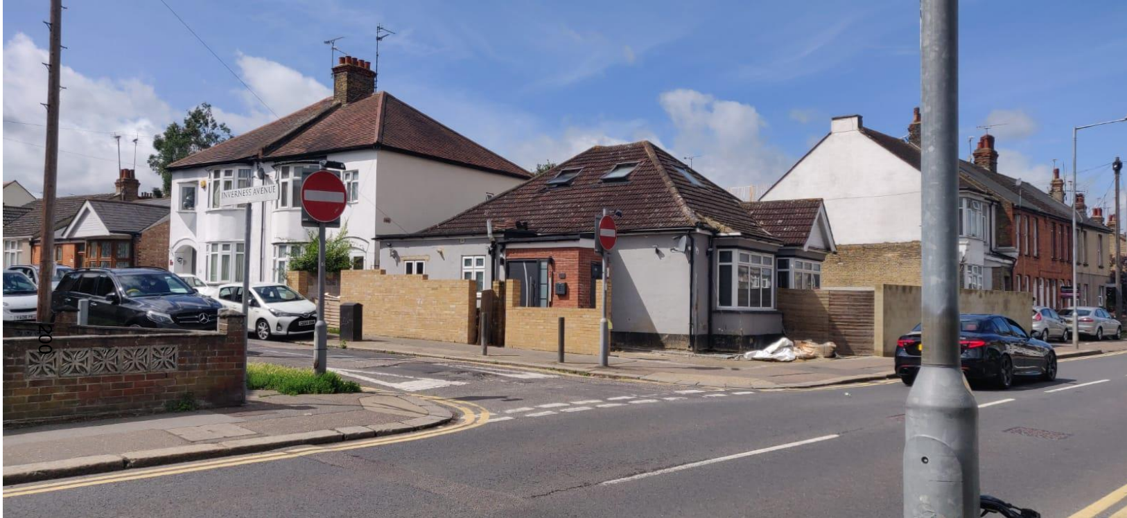
The site from Fairfax Drive showing the new boundary walls, porch and hardstanding
