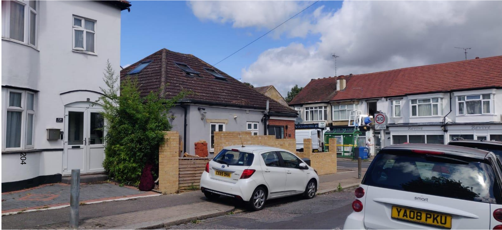
The boundary wall and porch along Inverness Avenue
