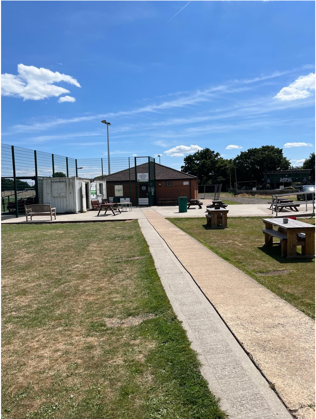
view to rear of site
